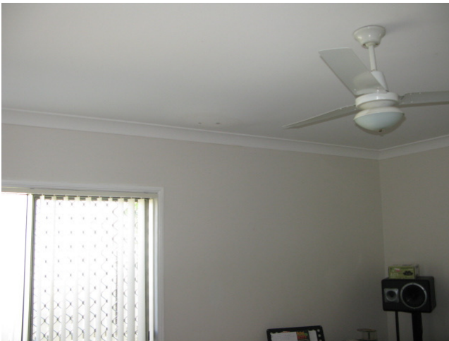
Picture 7 - downstairs wall of lounge room
