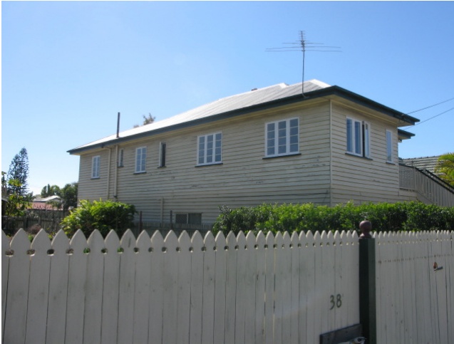
Picture 4 – western side weatherboard wall
