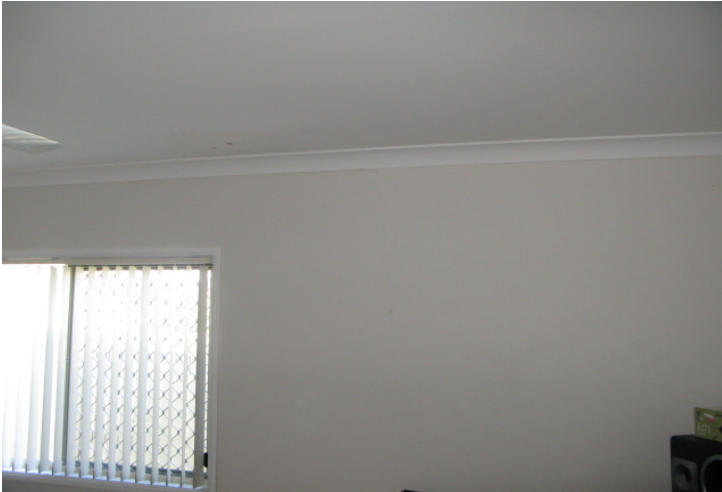
Picture 2- side wall of lounge room in the lower-level
